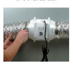
Attach the ducts with clamps.
